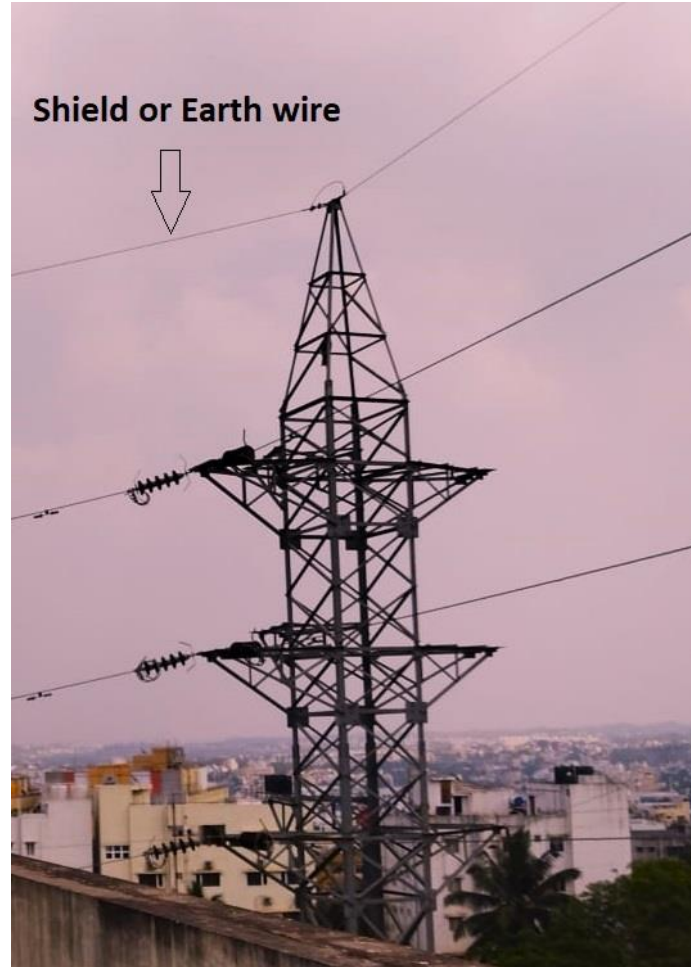
Figure 34. Shield or earth wires in transmission lines
