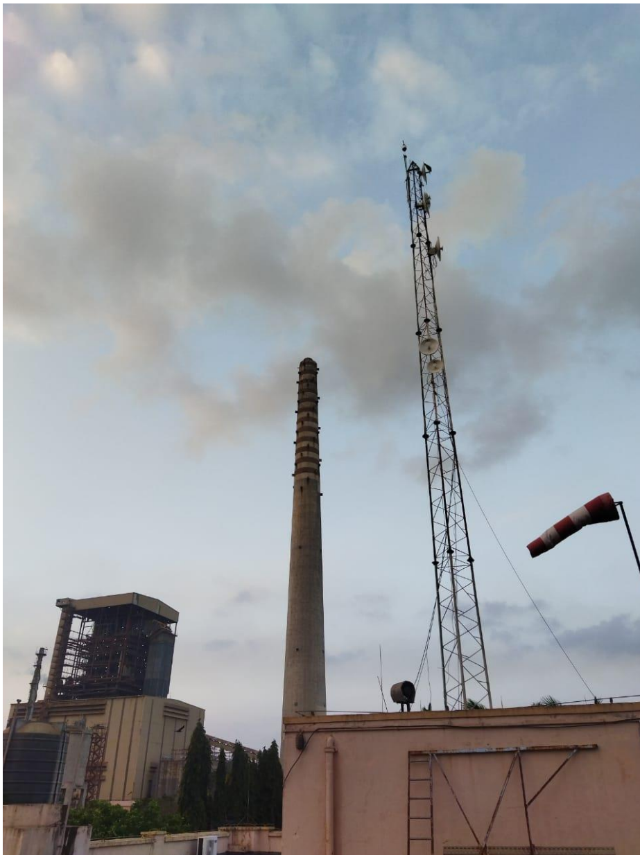
Figure 43. Telecommunication tower in building
