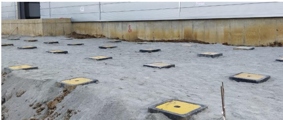
Figure 35. Multiple earth electrodes in parallel connection
