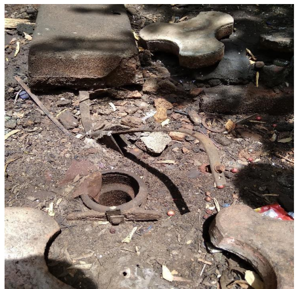
Figure 18. Improper maintenance of earth pits
