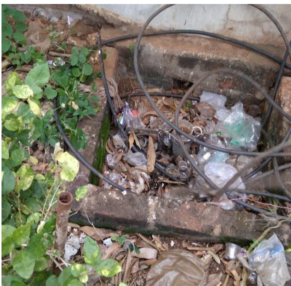
Figure 18. Improper maintenance of earth pits
